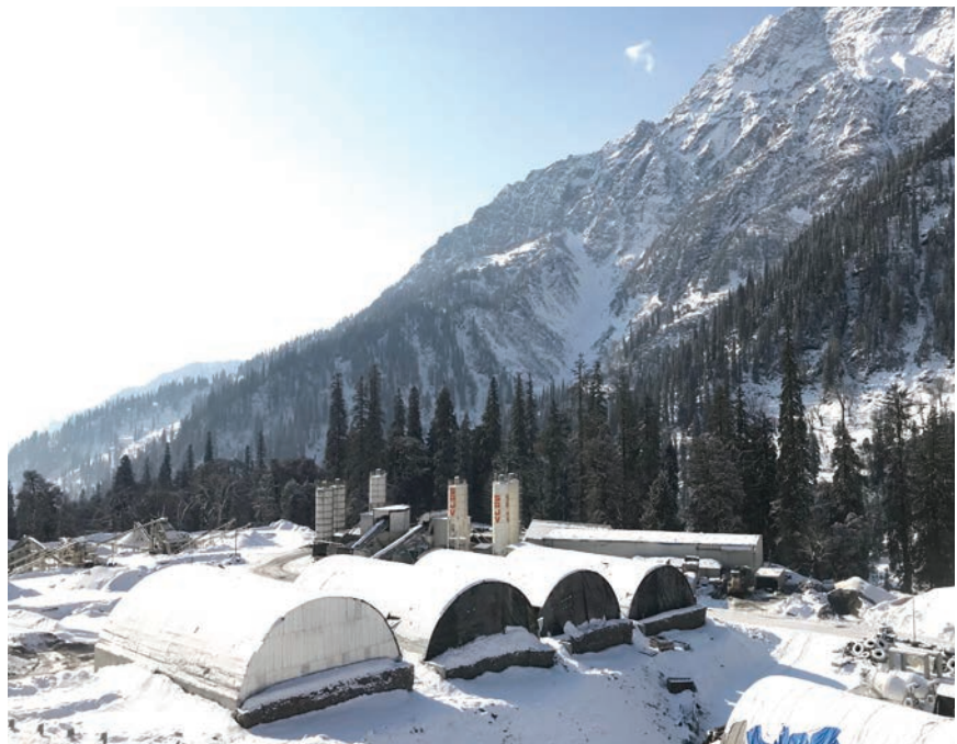
Part of construction site in January 2018
