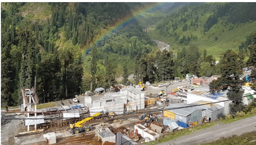
View of construction site near south portal of the tunnel
