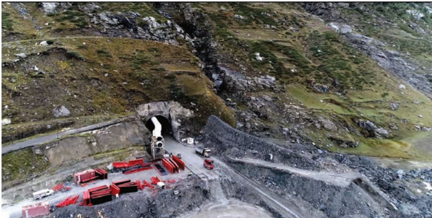
View of north portal of the Rohtang Tunnel
