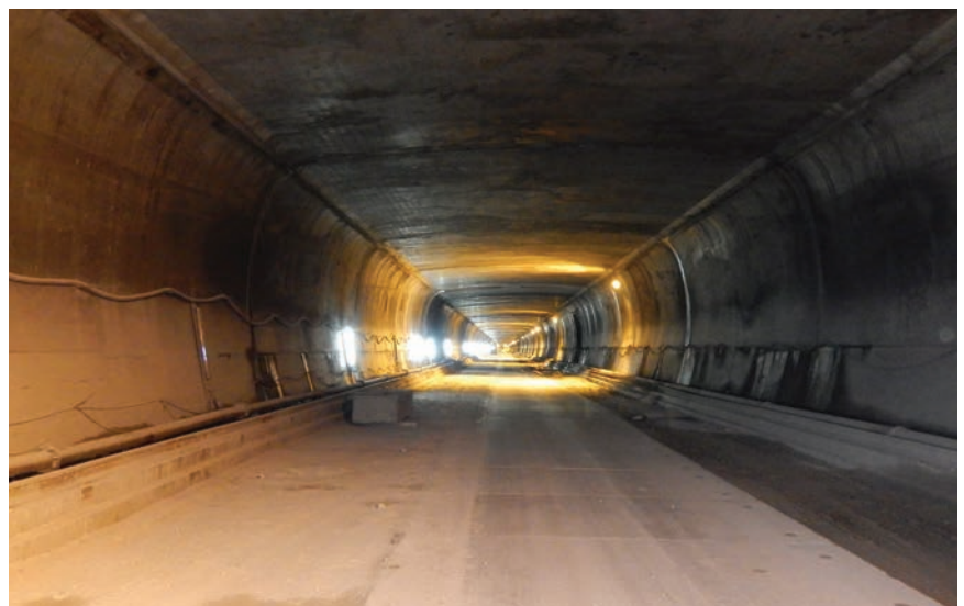
Tunnel photo taken in January 2018
