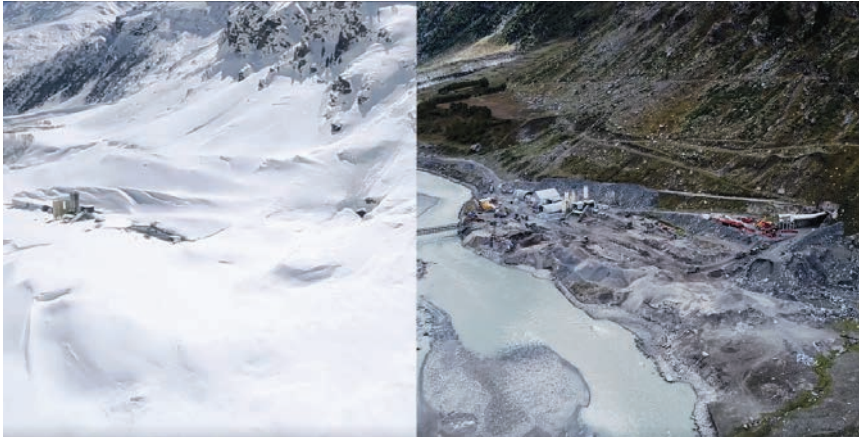
Construction site at north portal in winter (left) and summer (right)
