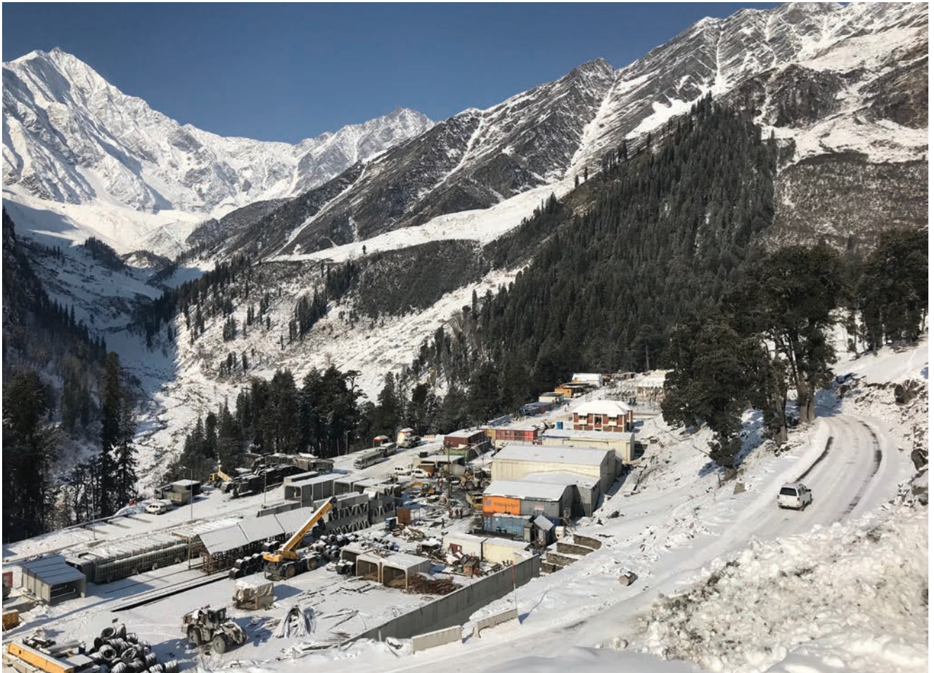
On-site precast-concrete plant
