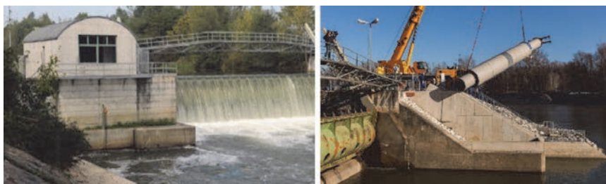
Figure 1. View of Retznei Barrage with the original hydropower plant (photo on the left) and the new hydropower plant with the tube-type double rotating screw on the left bank side (photo on the right)
