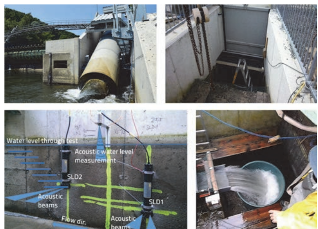
Figure 12. View of power screw from tail water (top left), view of intake channel towards head water, intake gate is closed (top right), mounting SLD probes and water level meter in intake channel and schematic illustration of the operating mode (bottom left), and filling gauging barrel with pumped water at the end of the fish trough (bottom right)
