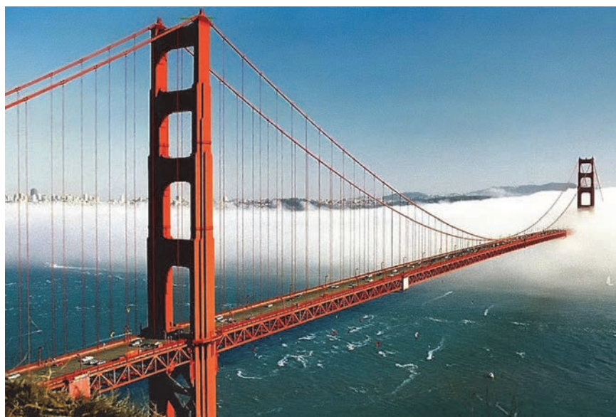
Figure 1. Corrosion protection – a never ending activity at the Golden Gate Bridge
