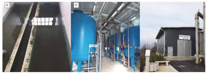
igure 3. Filters situated in Karašnica plant: a) gravity filter b) filters under pressure and facility accommodating these filters
