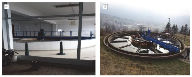
Figure 2. Circular settling tanks at Karašnica plant: (I) internal settling tank (T1) with a capacity of 50 I/s (II) external settling tank (T2) with a capacity of 100 I/s
