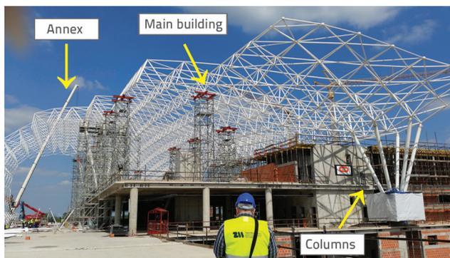
Figure 14. Characteristic new terminal segments in the construction phase
