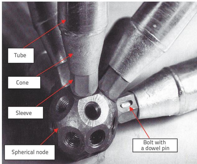
Figure 3. MERO system components - typical node [8]
