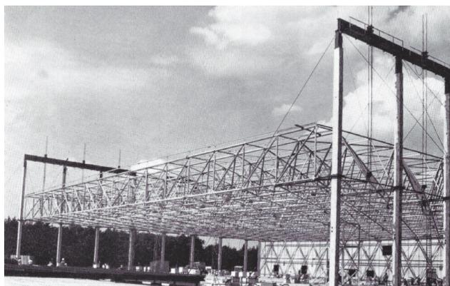
Figure 13. Erection of a fully assembled structure on supports [8]
