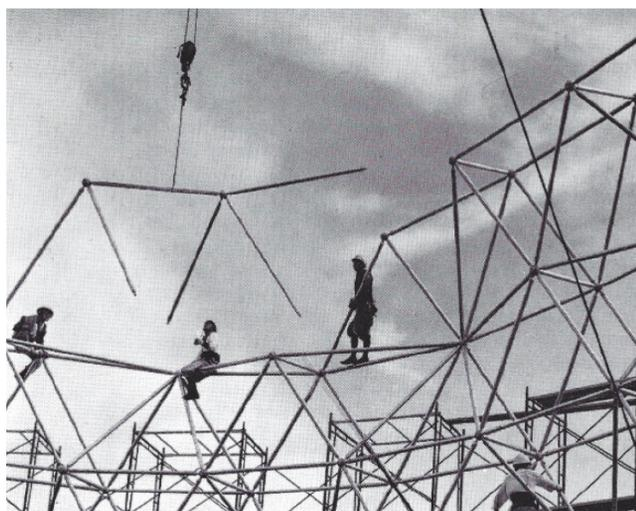
Figure 10. Free cantilevered assembly method [8]
