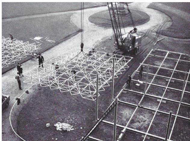
Figure 11. Erection of an assembled structure with crane [8]
