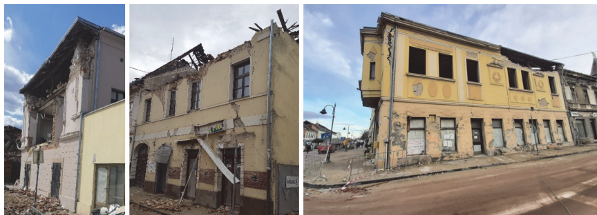
Figure 4. Façade wall mechanism [17]
