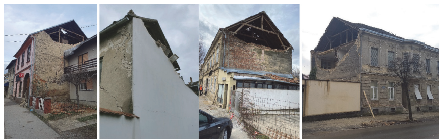
Figure 3. Gable wall mechanism [17]
