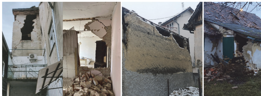
Figure 5. Mechanism of irregular geometry or atypical position [17]
