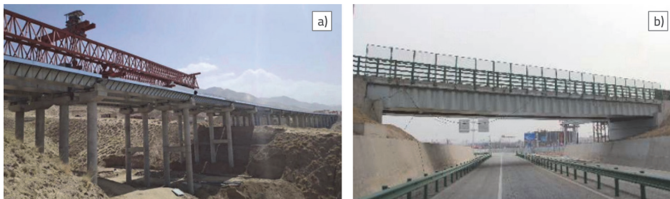
Figure 1. The construction and service state of composite box-girder bridges in China: a) The expressway bridge of Dunhuang to Dangiin mountain; b) The simply supported bridge at Jingzhong Airport
