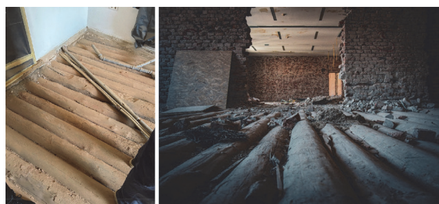
Figure 15. Floor structure made of three-side hewn beams in a residential building and a monumental structure
