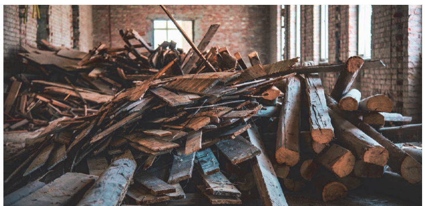
Figure 32. Dismantled timber primary load-bearing elements during structural rehabilitation
