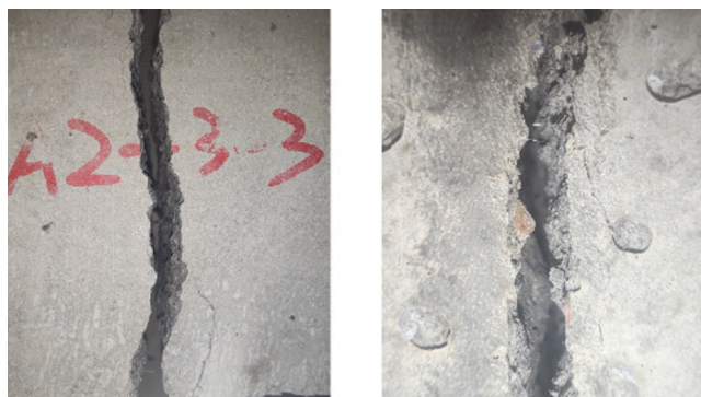
Figure 8. Splitting tensile failure surface of DSBFC
